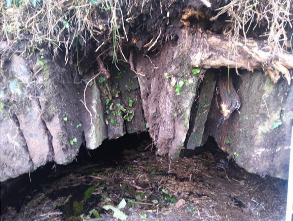
Collapsed sections of upstream arch
