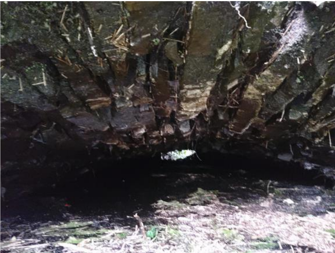
Missing masonry and collapsed soffit
